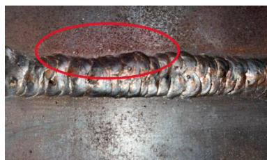
Figure 9. Welding Defects (Spatters) on Welding Workpieces (MIG) 2
